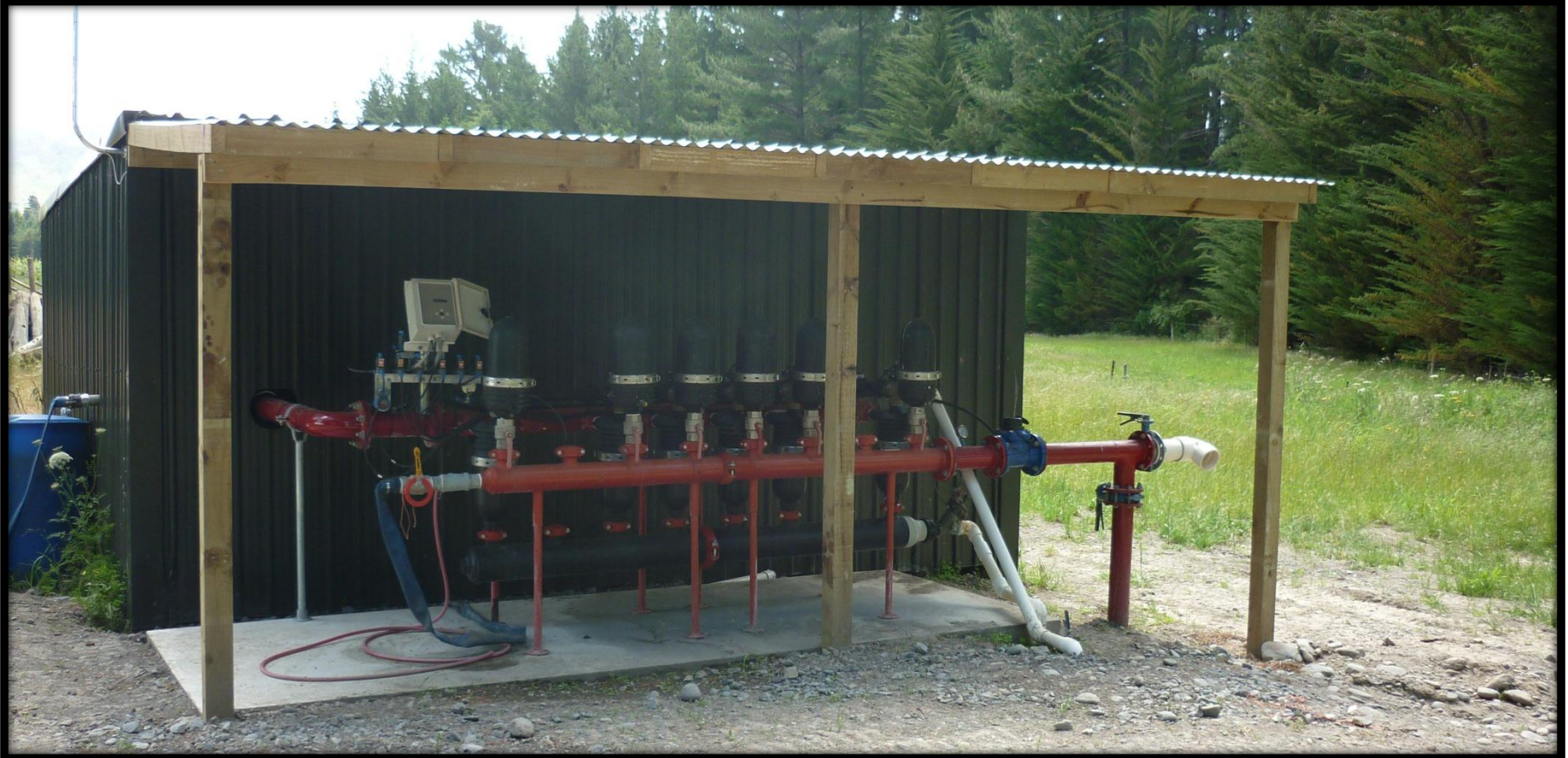
New Irrigation Filter System
