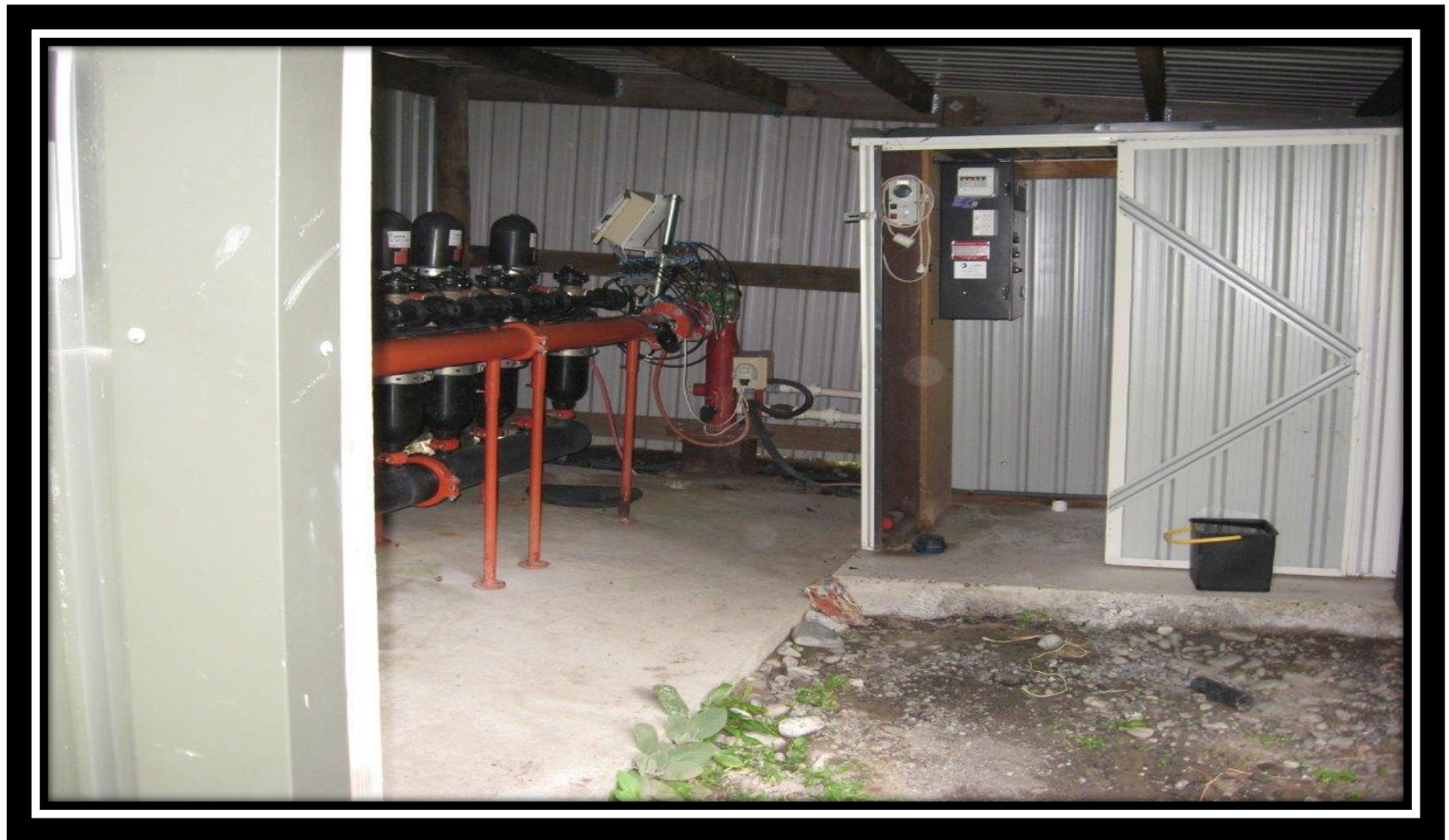
Earthquake Damage to Irrigation Headworks
